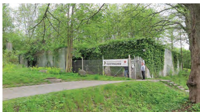
The exterior of the Ejby Air-Defence Bunker, built within the earlier Vestvolden. Nature is now adding its own coat of camouflage
